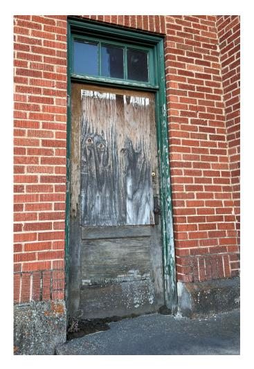
Item # 7 Entrance- South Door: Refurbish wood exterior transform and door. Door should be retrofitted with ADA handle. Reglaze and repair glass on 21 panes
